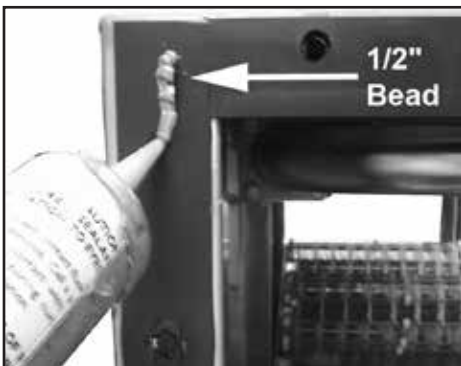
Fig. 2 - 1/2" Silicone Bead
