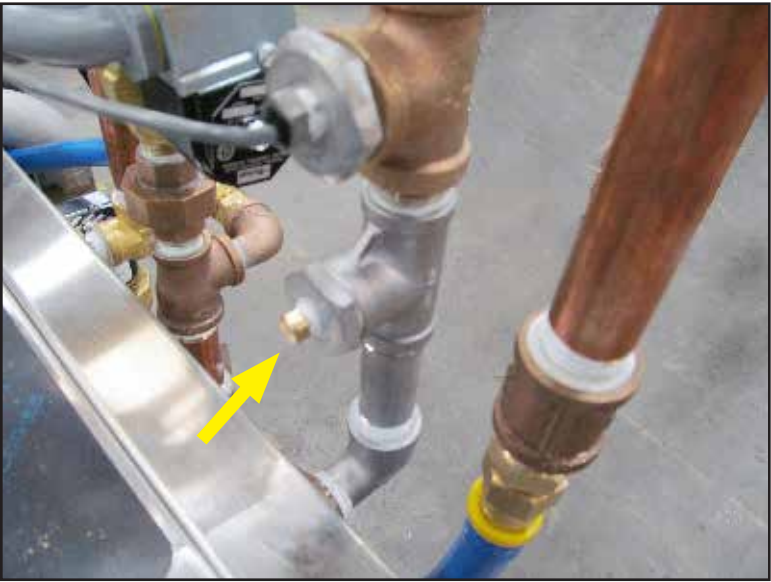
Fig. 33 - Rinse-aid injection point.
