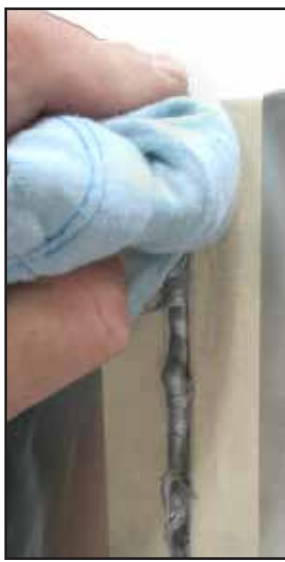
Fig. 13 - Smoothly remove excess sealant.
