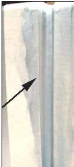
Fig. 14 - Remove masking tape.
