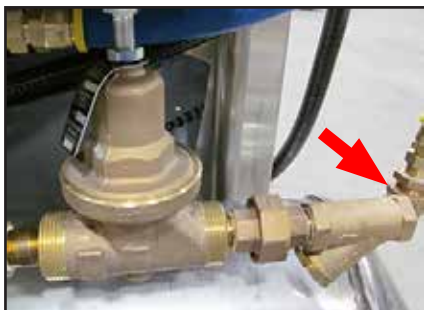
Fig. 8 - Standard and Heat Recovery hot water connection
