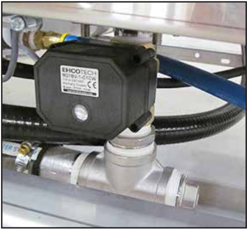
Fig.15 - Single tank drain connection
