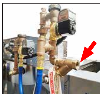
Fig. 9 - Hot water connection no internal booster
