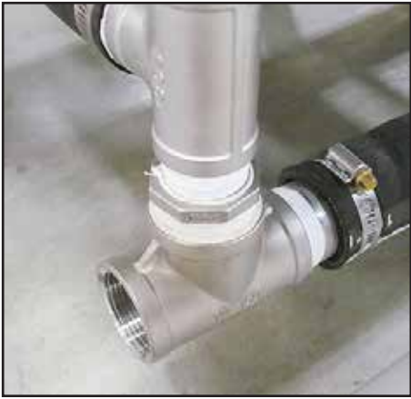
Fig.16 - Single tank with prewash drain connection
