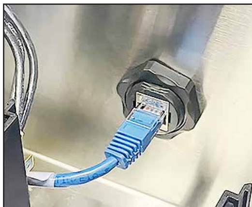
Fig. 4 - Ethernet port - Champion RJ45 from router (viewed from inside rear of control cabinet)
